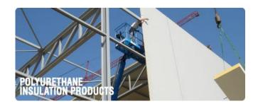
Insulated building panels are enjoying growth overseas due to their improved insulation performance and ease of construction. They are manufactured under factory controlled conditions utilizing a light weight insulation core sandwiched between two facing materials making insulated panels lightweight, quick to erect and free from problems of compression shrinkage and cold bridging associated with other forms of construction. Production of insulated panels may be continuous or discontinuous.
