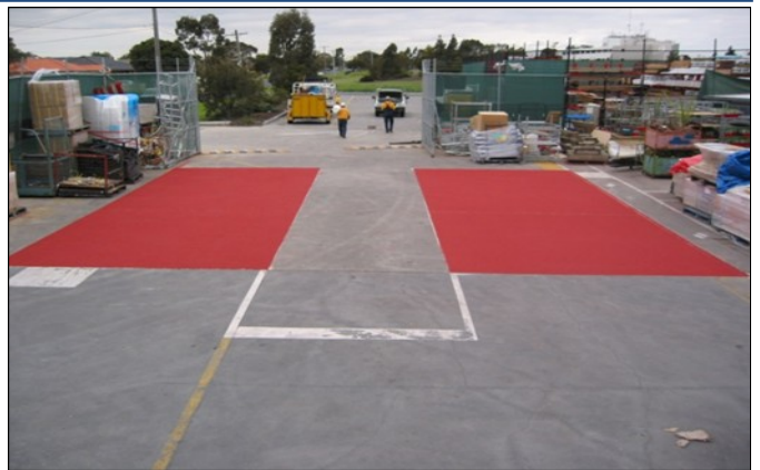
Bunnings Loading Dock
